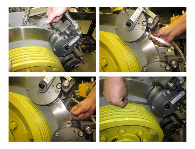
Figures 17: Check Brake Gap at 4 places around the brake to understand completely the brake position.
