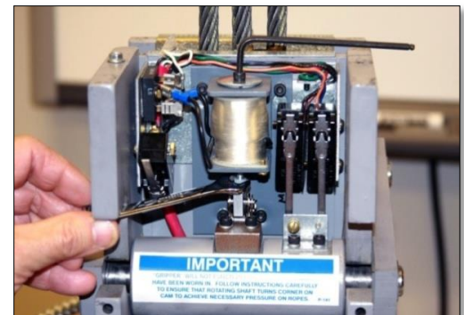
Figure 6: Brass Nut & Allen Screw Location
