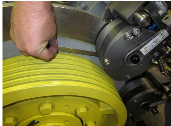
Figure 17: Check Brake Gap at 4 places around the brake to understand completely the brake position.
