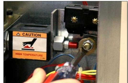
Figure 4: Turn Cam to Manual Mode
