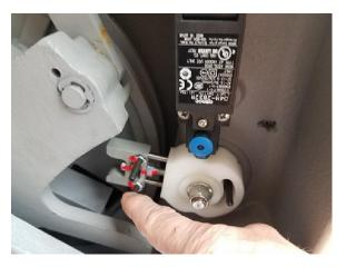
3. Pull the blue manual reset button on the over-speed switch to reset the switch.
